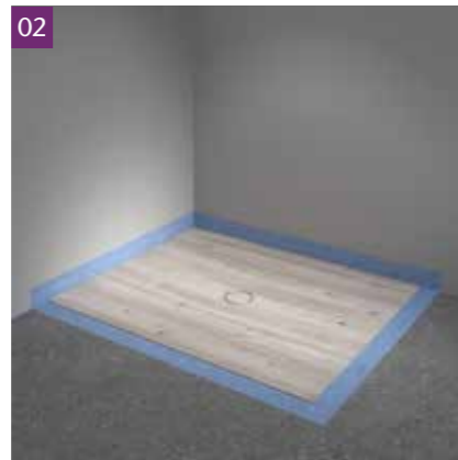
Fig. 2: Profi-Flex adhesive is used for bonding.
